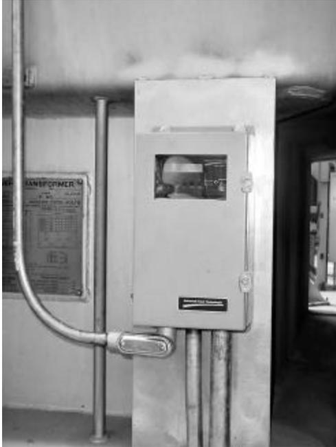
From here, programming can be done and readings made as needed. Also, connections to the station SCADA or other instrumentation via common protocols or current loop will be made in this location.
