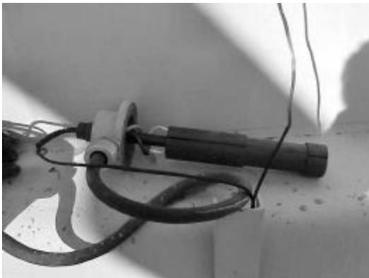
This assembly is then inserted into the well in the transformer top oil. In some designs, the heating element is actually part of the well and cannot be removed separately.
